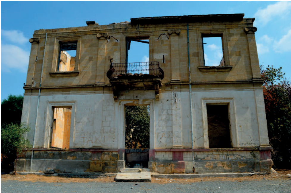
Figure 16. A house in the UN buffer zone, Nicosia.
